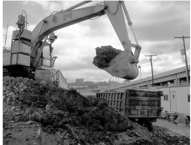
Figure 16. Typical dig for truck loading.
