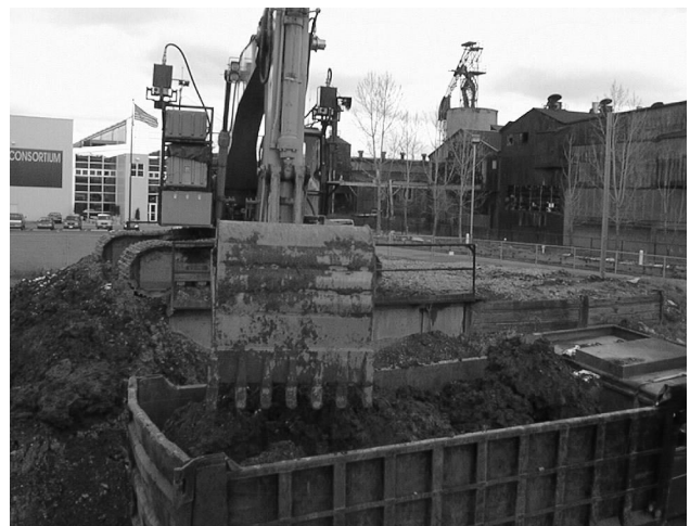
Figure 17. Truck is loaded after six passes.
